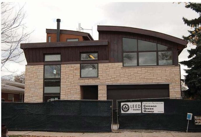
Reclaimed copper roof, gutters and fascia ▪ Thermostat on front windows operates motorized blinds for energy efficiency in summer & winter
