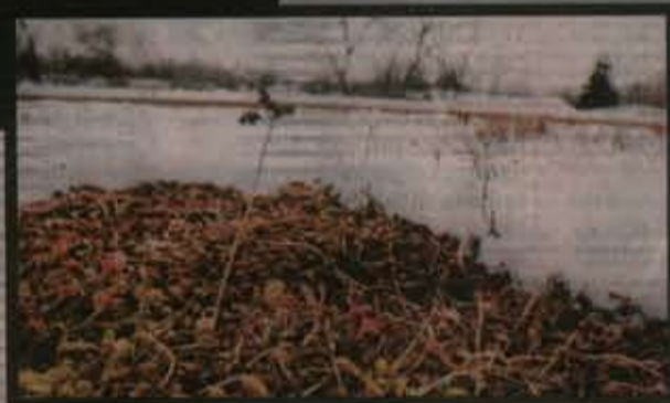
The green roof is made of several inches of topsoil, grass and a variety of flowering plants for water retention.
